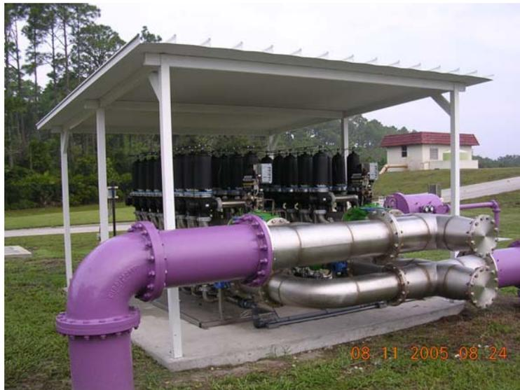
Custom Type 316 stainless steel manifolding fabricated by Miller-Leaman to accommodate future expansion of the *Turbo-Disc Filter* system
