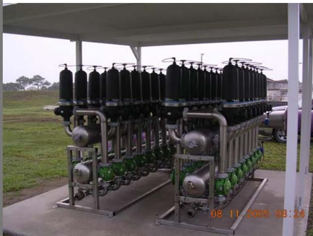
*Miller-Leaman’s automatic Turbo-Disc Filter system installed at Dunes Utilities; current filtration capacity is approximately 4,500 GPM*
