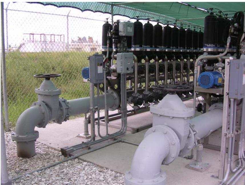
*Intake Water Piping to Turbo-Disc System with Booster Pumps*
