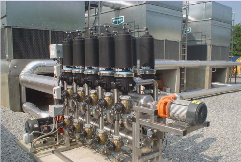
1,000 GPM Turbo-Disc Filter Side-Stream Skid System
