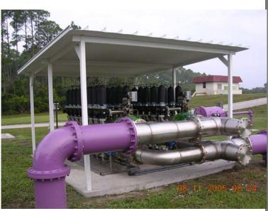
Custom Type 316 stainless steel manifolding fabricated by Miller-Leaman to accommodate future expansion of the Turbo-Disc Filter system
