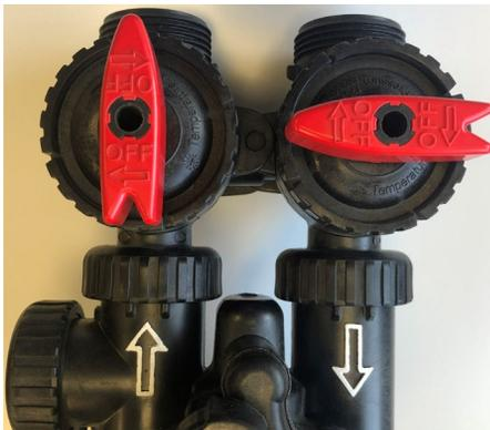
**STEP 2-** Shut off the incoming water supply using the Carbon Filter Bypass as shown in Picture
