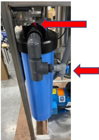
**STEP 3-** Relieve Pressure from Filter Housing using The ¼” Test Port or the “Red” button on top of the Filter Housing Cap
