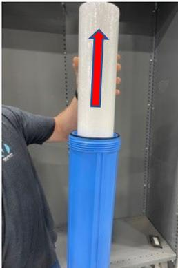
**STEP 5- REMOVE OLD FILTER AND RINSE OUT FILTER HOUSING OF ANY DEBRIS**
